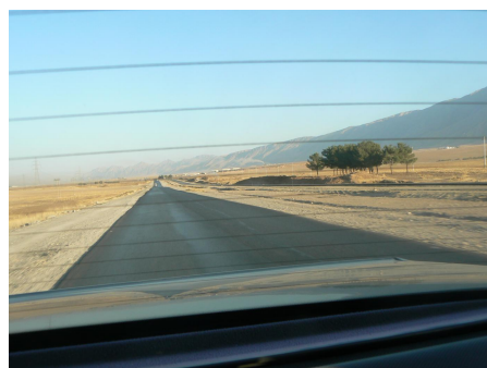
Newly asphalted road Dukan-Sulaymaniyah. New lanes being built.
